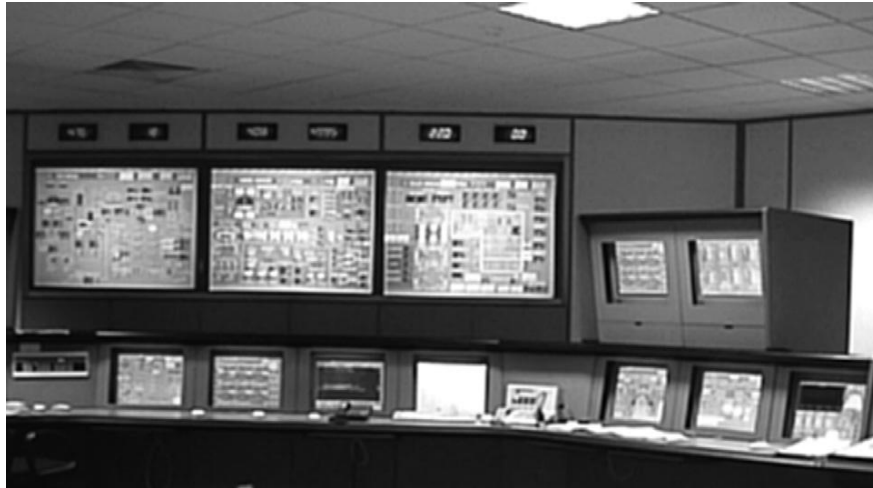
FIGURE 32.13 Monitors in the control room of an electricity generating station display the outputs from numerous measurement systems.
