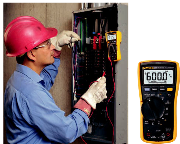
Figure 1-11 Testing for the presence of voltage. Photos courtesy Fluke, www.fluke.com . Reproduced with Permission.
